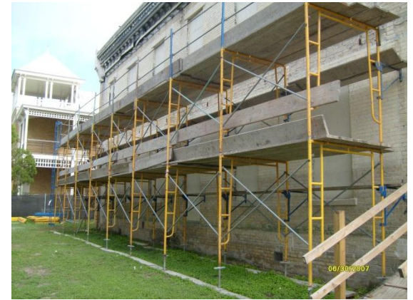
Masonry Restoration – BLDG 601 & 602 Fort Sam Houston
